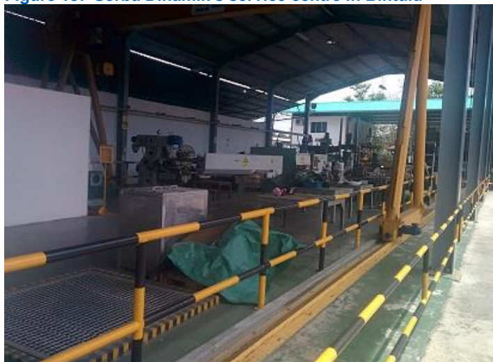
Figure 13: Serba Dinamik's service centre in Bintulu
