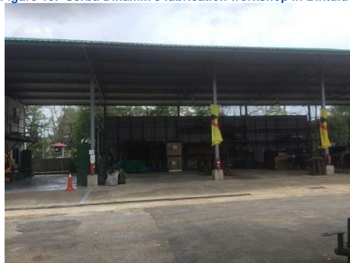
Figure 16: Serba Dinamik's fabrication workshop in Bintulu
